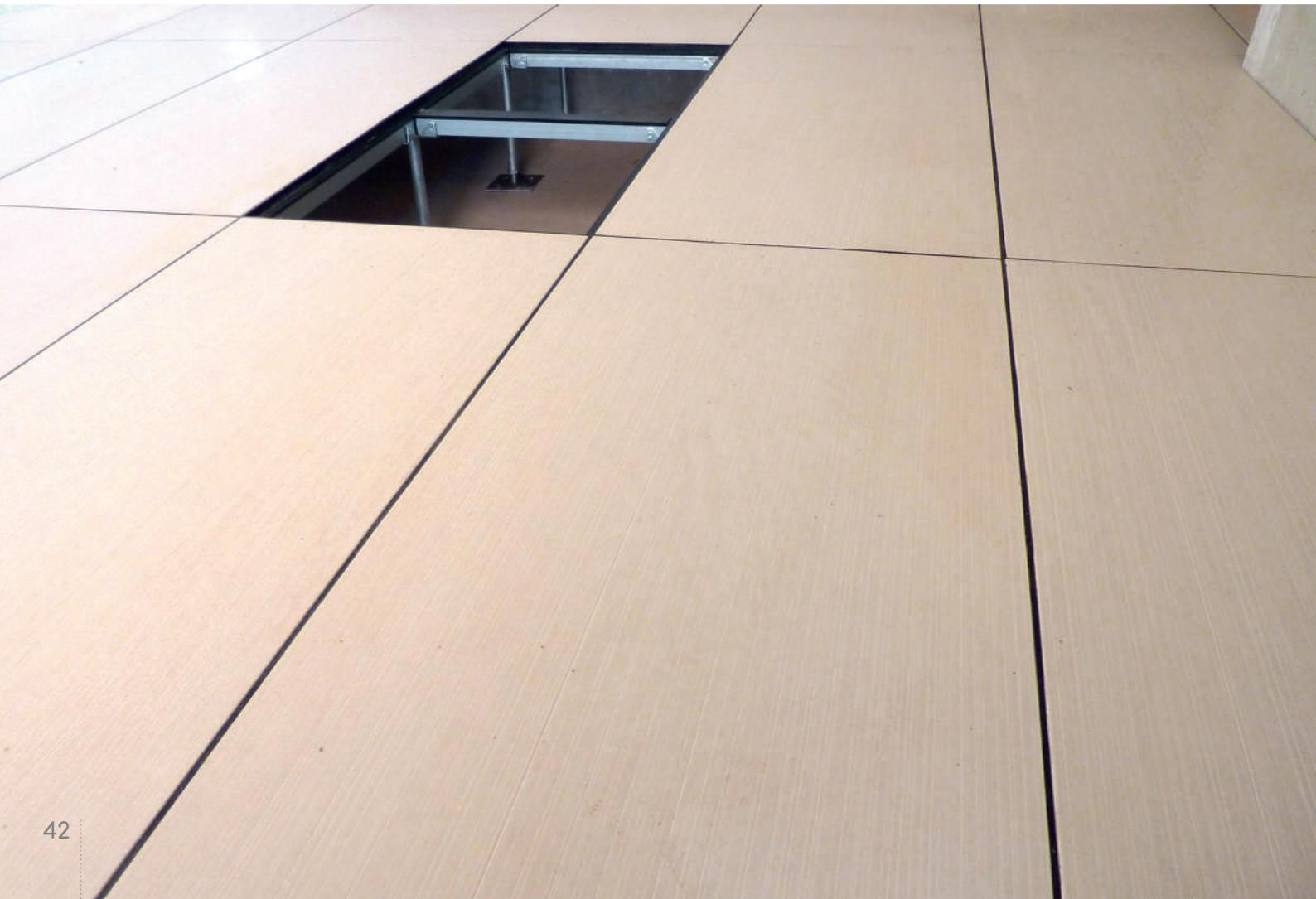
WANDEFLOOR INWASE is a new ceramic raised floor system for interior spaces, up to four times lighter than traditional solutions.
