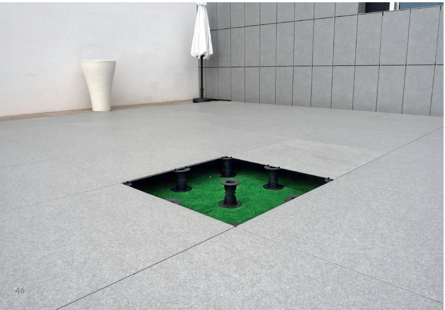
Wandefloor Outwase, is a new raised floor solution for outdoor spaces, up to four times lighter than a traditional raised flooring. The application of Wandeslim reinforcement allows this solution to reach a very high mechanical resistance, which guarantees safety and allowing its installation on terraces, parks or common areas.
